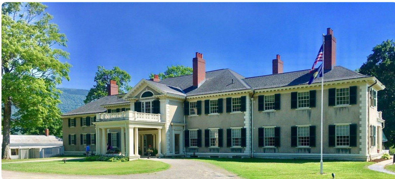
Figure 3a. A photograph of the Hildene House as viewed from outside the structure
